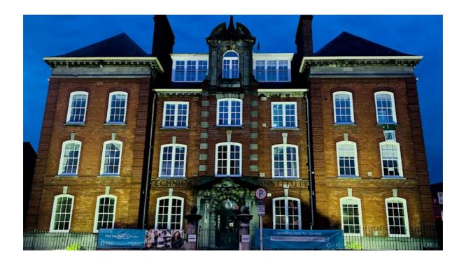
Project partners TUS and LCETB met at the Demo building in Limerick in November to establish a timeline of works and identify test areas for the installation of insulation panels. LCETB organised the drilling of boreholes on this day to identify the building typology. It was confirmed that the building is made from mass concrete and has reinforced beams in the ceiling. This timeline of works is now being closely monitored during fortnightly meetings between project partners TUS and LCETB.
